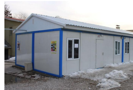
Typical accommodation unit, materials on site
