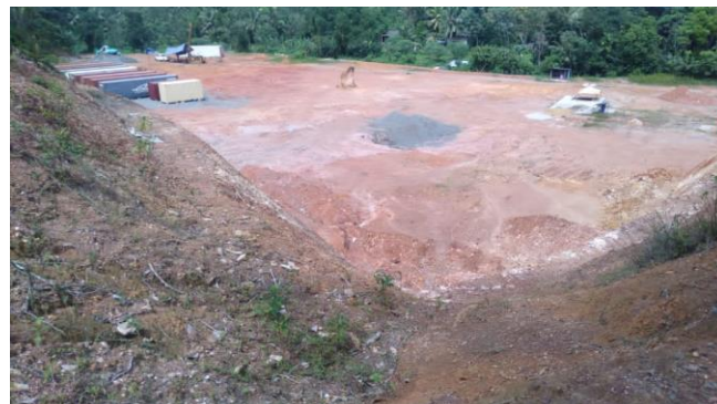
Site clearing commenced January 2020
