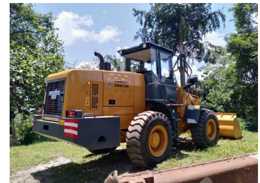
New IT loader on site
